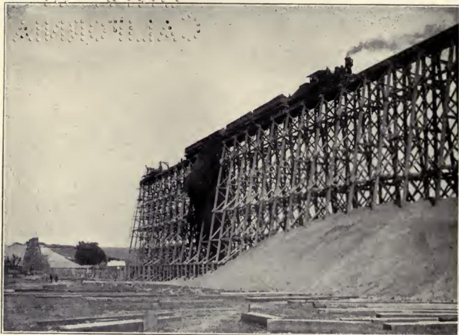
THE MAKING OF AN EMBANKMENT BY DUMP-TRAIN
